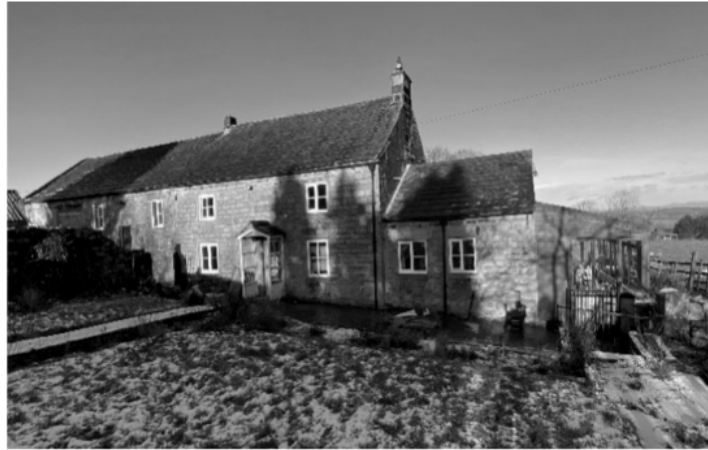
Figure 1: External View of Farmhouse
