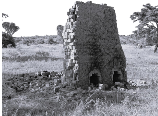
Figure 1: A double-chamber clamp kiln brick stack (Source: Authors' fieldwork)
