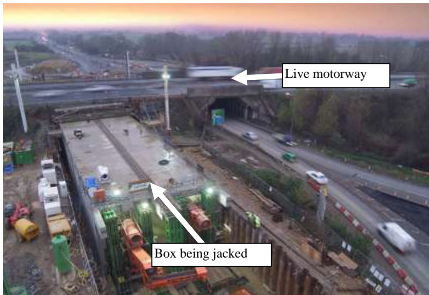
Figure 1. RC Box-Jacking under a live motorway
