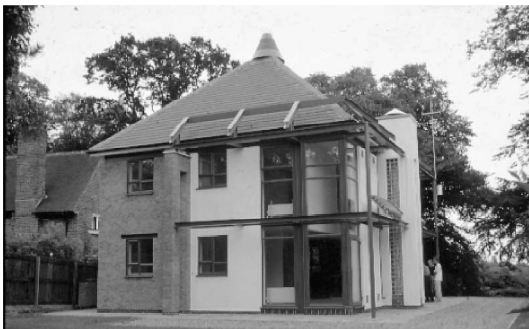
Figure 1: BIPV, Eco Energy House [EEH] (University of Nottingham, UK)
