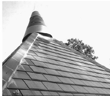
Figure 2: EEH PV slates integration Figure 3: Roof View – EEH
