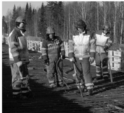
Figure 2. a) Hand-arm vibration gauge, attached to a working glove. b) Workers vibrating the concrete slab, having the poker vibrators approximately 1 meter from the ears
