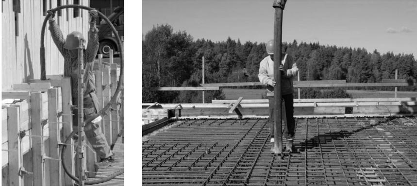
Figure 1. a) Work posture when compacting NVC in wall structures. b) Casting of SCC on slab
