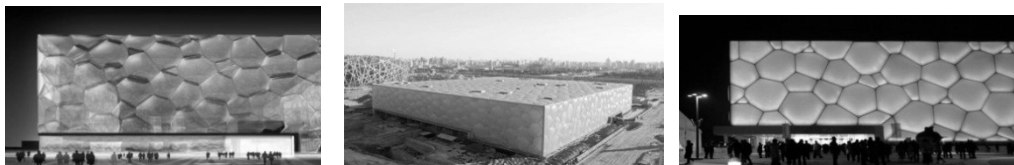
(a) The design vision (b) During construction (c) The constructed facility
