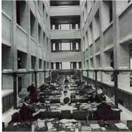
Figure 1: Inside the Larkin Building, New York 1904
