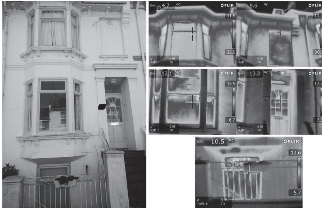
Figure 4: Typical photo of house and corresponding thermal images
