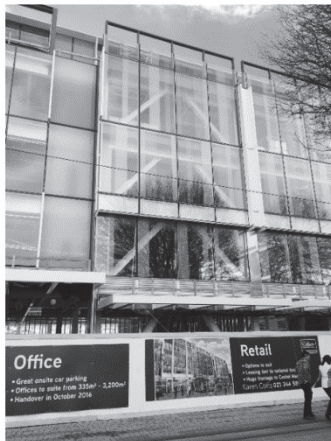
Figure 3: Like many new buildings, the steel structure is clearly expressed in the facade design.
