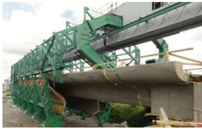
Figure 5: MSS applied for the construction of the bridge deck sections
