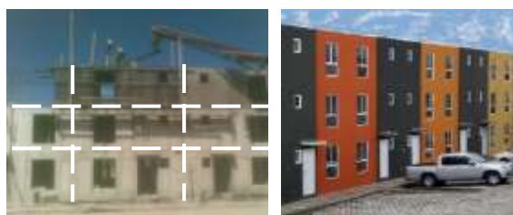
Figure 2: Standardized concrete segments applied at Victoria
