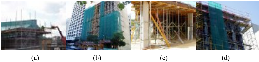
Figure 4: Safe construction practice images
