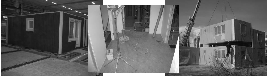
Figure 2: Prefabrication and site assembly of volumes including finishing.
