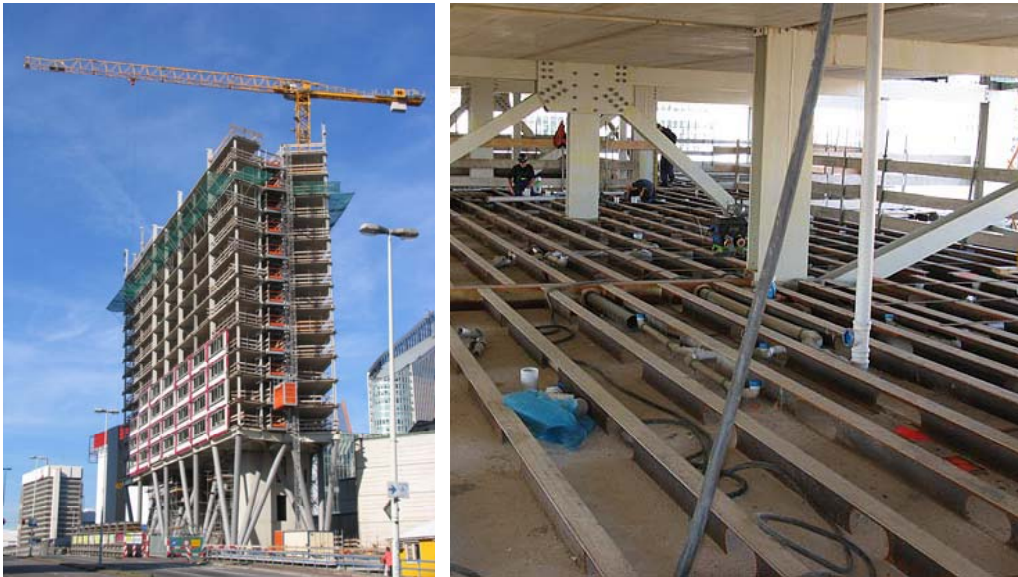
Figure 9: La Fenêtre, The Hague the Netherlands
