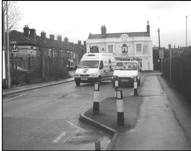
Figure 9: Photo of Pinch Point
