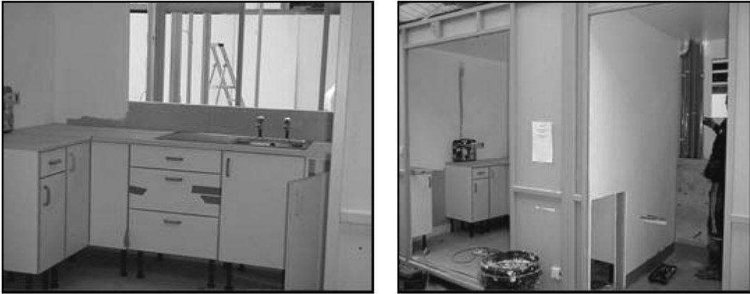
Figures 6 and 7: Pods being Fitted-out
