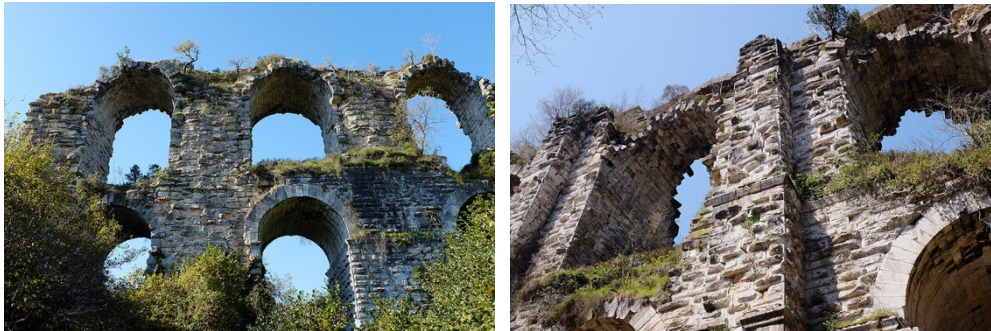
Figure 2 Kumarlidere (L) and Kurşunlugerme (R) aqueduct bridges (Photos: Smith 2015)
