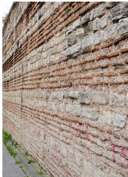
Figure 5 'Opus vittatum' construction – alternating courses of stone and brick. (Photo: Smith 2014)
